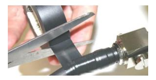
**Note:** To make a strong watertight connection, keep a high level of tension in the butyl mastic when you stretch it over the cable and connector.
