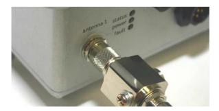
4. Wrap a layer of electrical tape (sticky side out) over the arrestor to node connector and wrap approximately 2.5 cm (1 inch) of cable. Overlap the tape by 40% with each turn.
