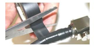
**Note**: To make a watertight connection, keep tension in the butyl mastic when you stretch it over the cable and connector.
