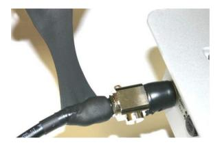
7. Wrap a layer of electrical tape (smooth side out, sticky side in) over the mastic tape.
