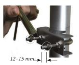
U-bolt\* mounted on pole—note addition of secondary nuts (circled) to meet 12–15 mm bolt length required by the universal mounting bracket.
