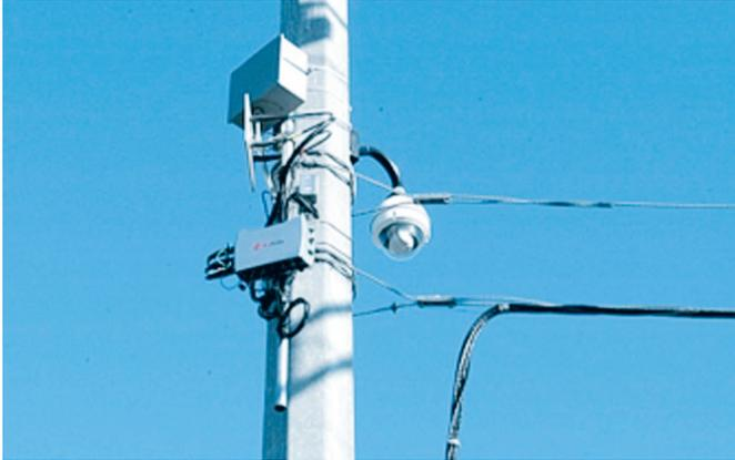
*Video Surveillance Camera Connected to Firetide Wireless Mesh Node*
