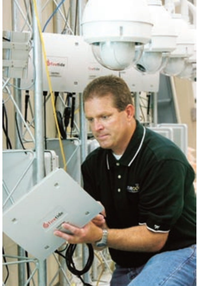
Preparing for the installation
