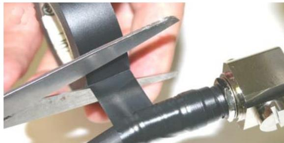
**Note:** To make a strong watertight connection, keep a high level of tension in the butyl mastic when you stretch it over the cable and connector.
