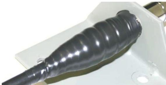
8. Wrap a second layer of electrical tape over the first layer of electrical tape.
