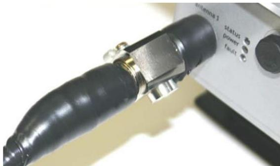
7. Wrap a second layer of electrical tape over the first layer of electrical tape. The lightning arrestor connections are ready for installation in an outdoor environment.
